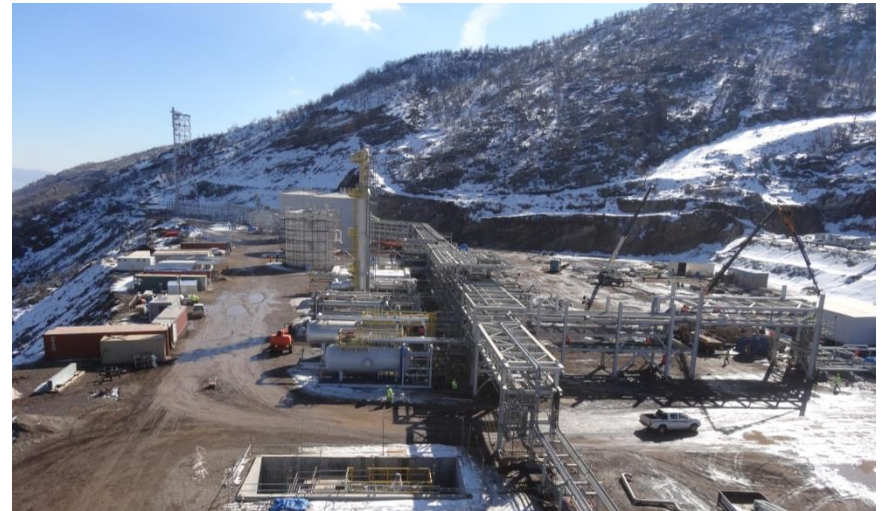
Above: Progress at the 30,000 barrel per day Phase 1 production facility
